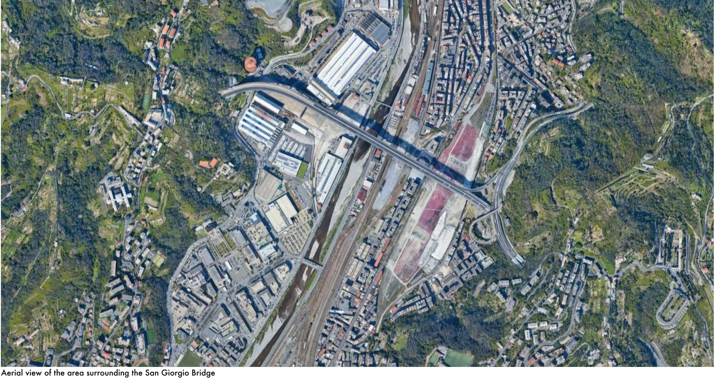
Aerial view of the area surrounding the San Giorgio Bridge
